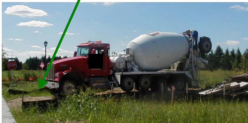
Designated Concrete Washout Areas with a Rock Entrance
