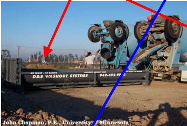
Designated Concrete Washout Bin
